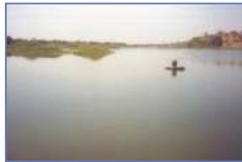
Dapora Dam, MJP Water Supply, Jalgoan City Maharashtra 2001 - 41% saving
