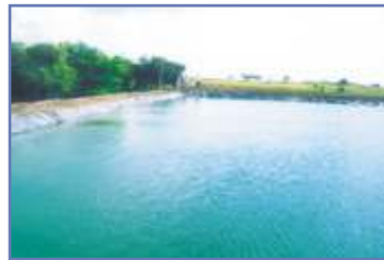
Industrial Water Tank Hospet, Karnataka
