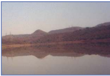
Nilona Dam, Water Supply, Yavatmal City Maharashtra 2005 - 39% saving
